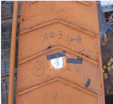
Figure 4. Strain measurement point on cantilever
